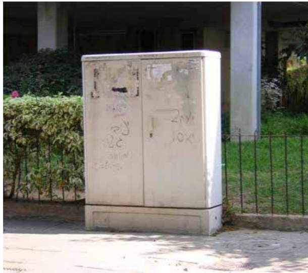
Electric Feeder Pillar Placed on Footpath, Delhi (Source: ) https://exceedingsky.wordpress.com/2012/06/25/coolest-street-electrical-box-graffiti/
