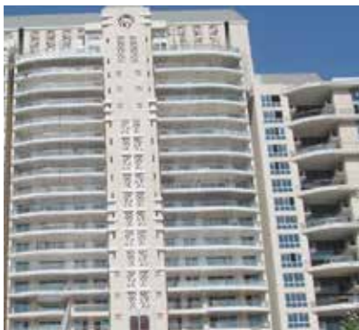
Shafts Enclosed by GRC Jali, EMAAR, Gurgaon (Source: ) http://www.maheshgrc.com/Multi_Story_Housing.html
