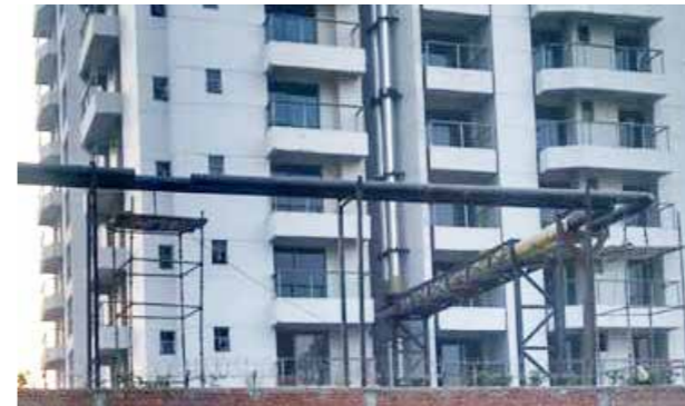
DG Set Stack Concealing, Paras Dews, Gurgaon (Source: ) Author
