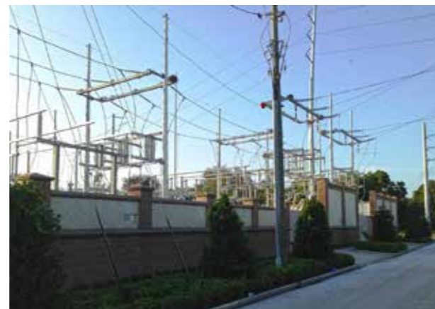
Architecturally Treated Boundary Wall, Substation-Florida (Source: ) http://www.kam-services.com/new-gallery-2/
