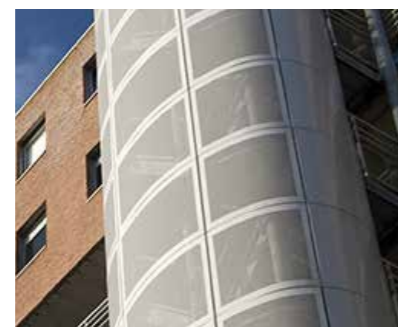
Perforated Metal to Screen Utilities (Source: ) https://www.johnroccosales.com/news-blog/2015/9/10/architects-top-5-advantages-of-perforated-metal
