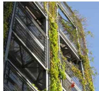
Vertical Greens to Screen Utilities (Source: ) http://www.aucklanddesignmanual.co.nz/sites-and-buildings/mixed-use/guidance/thebuilding/facadedesign
