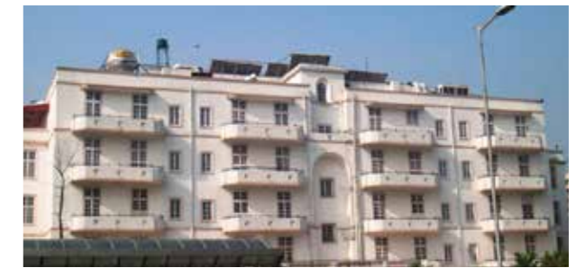
Exposed Rooftop Equipments, Hotel Ambassador, Khan Market, New Delhi (Source: ) http://thistimethatime.blogspot.com/2012/10/182-khan-market.html
