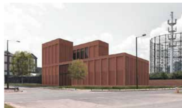
Red Brick Clad Electric Substation, Greenwich Peninsula (Source: ) http://www.greenpen.london/blog/electricity-substation
