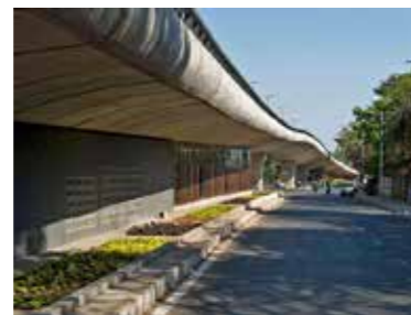
Space under Flyover, IIM A-Vastrapur Flyover, Ahmedabad
