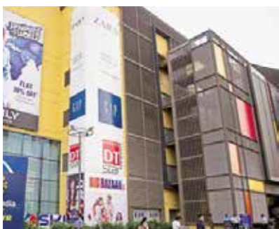
Screening Utilities and Staircases (Source: ) http://www.theglobalrealty.com/2019/08/04/dif-transfers-noida-mall-land-to-jv-firm-reduces-dues-to-rs-5500-0/architects-top-5-advantages-of-perforated-metal
