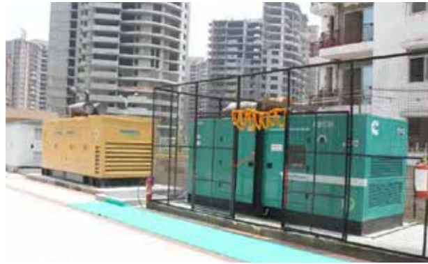
Exposed DG Set, Victory Crossroads, Noida (Source: ) https://www.hindustantimes.com/noida/in-a-first-noida-high-rise-to-run-diesel-gensets-on-png-fuel/story-mMmPUjRiu9TC1cnerEhHbN.html
