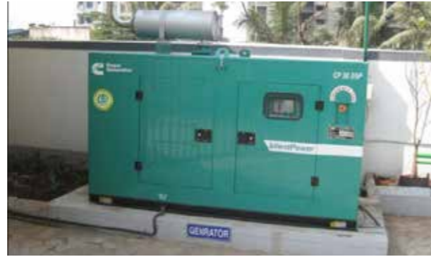
DG Set Along Compound Wall (Source: ) http://www.sudhirpower.com/DG_Set_Installation_Guide.pdf
