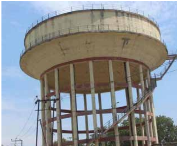
Ill-Maintained Service Reservoir (Source: ) http://tanknwon.us/water-tank-construction/
