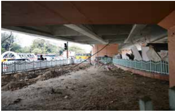
Unused spaces leading to dumping of garbage
