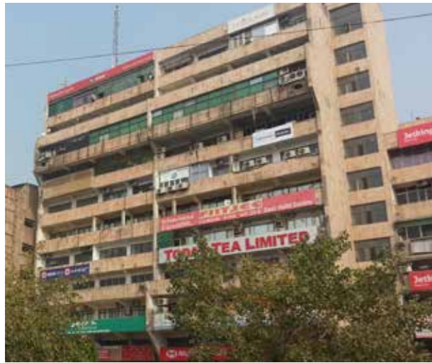
Exposed Outdoor Units in Elevation, Laxmi Nagar (Source: ) http://www.delhirealestateguy.com/wp-content/uploads/2015/11/20151104_134657.jpg
