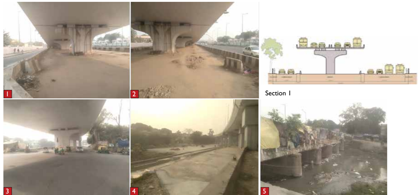
The underside of the flyover lying dysfunctional and underutilized
