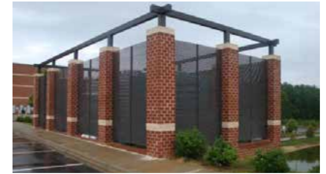
On Ground Utility Screening By Louvers (Source: ) https://www.ametco.com/spotlight/
