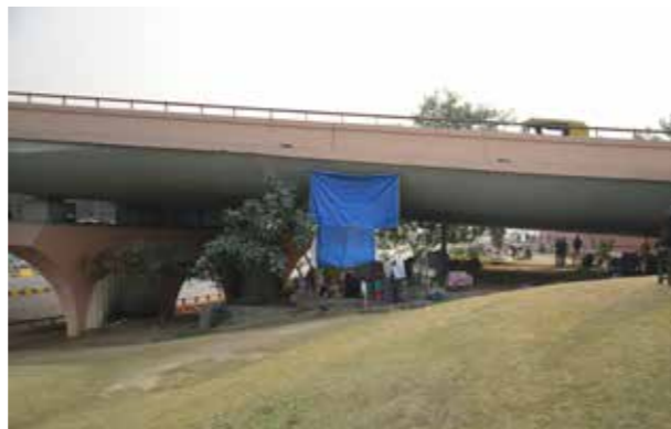
Encroached as shelters by homeless
