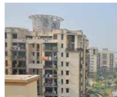
Purvanchal Silver City, Noida (Source: ) http://www.purvanchalconstruction.com/silvercity-features.html
